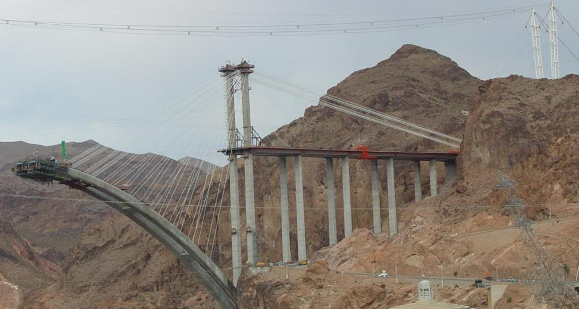
**Note steel X-Bracing installed between arches at segments 6 & 12. Steel X-Bracing is in the process of being installed between the 18<sup>th</sup> segments. Note the work platform is already installed.**
