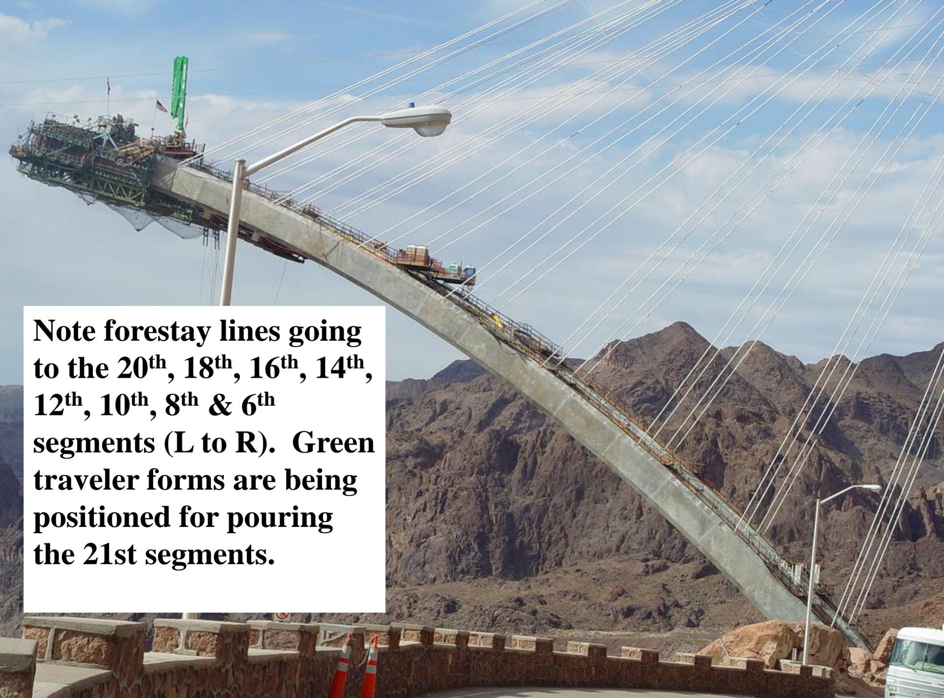
**Note forestay lines going to the 20<sup>th</sup>, 18<sup>th</sup>, 16<sup>th</sup>, 14<sup>th</sup>, 12<sup>th</sup>, 10<sup>th</sup>, 8<sup>th</sup> & 6<sup>th</sup> segments (L to R). Green traveler forms are being positioned for pouring the 21st segments.**
